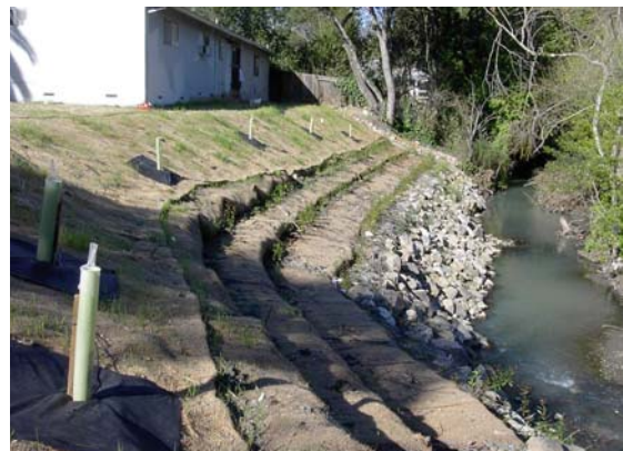
Completed stream bank stabilization with willow emergence March 2008.
