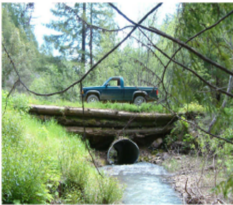
UPSTREAM OF UNDERSIZED CULVERT AND LOG JAM AT THE QUARRY BRIDGE SITE STREAM CROSSING WATER VELOCITY IN MAY 2003 IS RELATIVELY RAPID.
